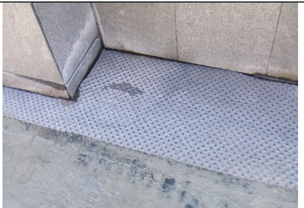
8. Drainage cell fabric under the tiling screed makes it easy to direct subterranean water to designated outlets.
