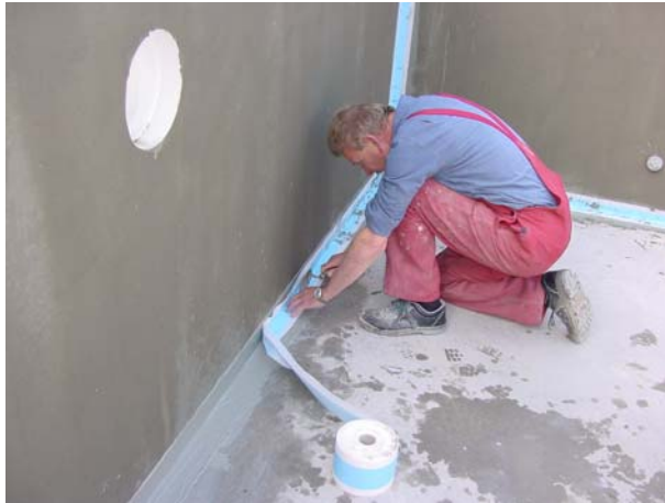
Image 4: Application of waterproofing tape to the fresh liquid applied waterproofing.
